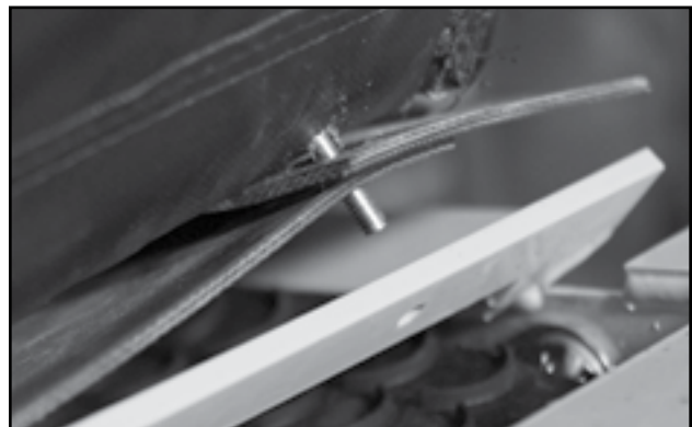
Fig 89 - Insert bolt through top, side and tail flashing
