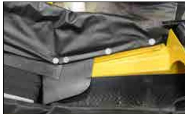
Fig 104 - Transition corner flashing in place
