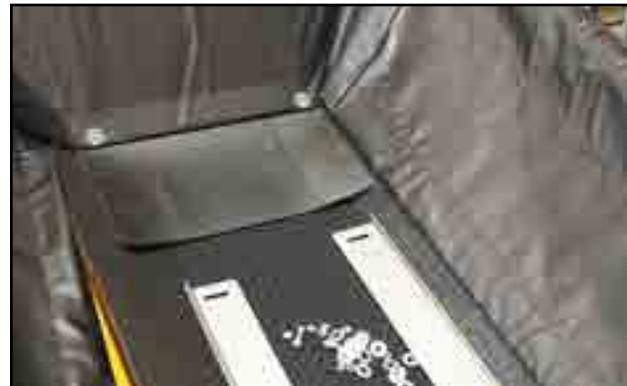
Fig 103 - Tail flashing on top of side flashing
