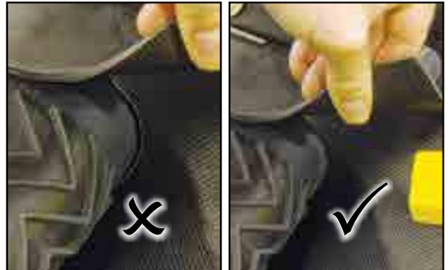
Fig 93 - Corner flashing must fit tight around the belt
