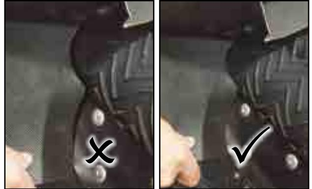
Fig 108 - Corner flashing must fit tight
