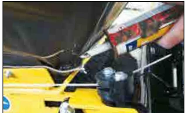
Fig 110 - Silicone gap in front corners
