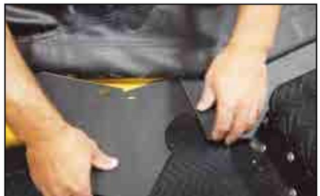
Fig 102 - Transition, Corner flashing
