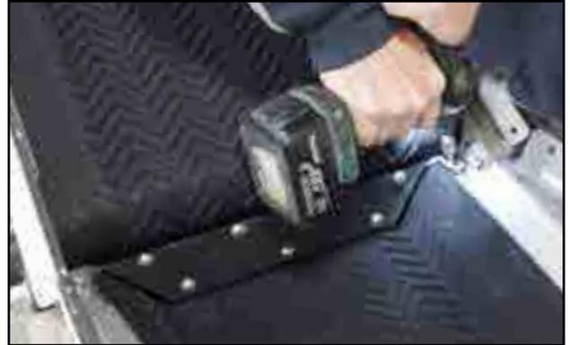
Fig 99 - Fasten transition flashing
