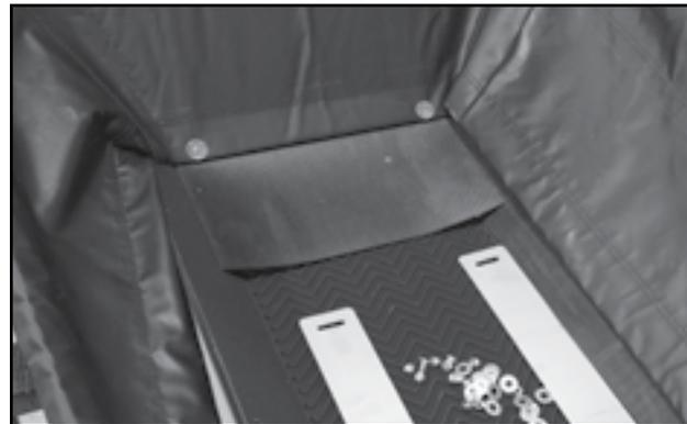
Fig 74 - Tail flashing on top of side flashing
