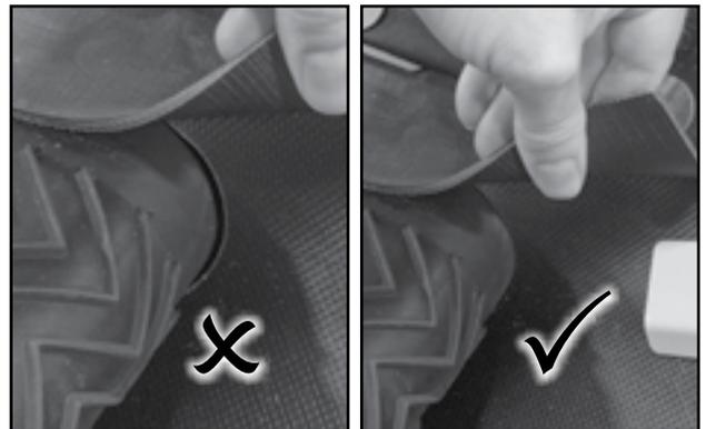
Fig 77 - Corner flashing must fit tight around the belt
