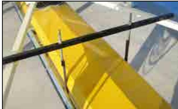
Fig 16 - Hanger bar with brackets bolted on
