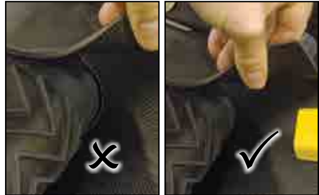
Fig 67 - Corner flashing must fit tight around the belt
