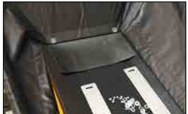
Fig 64 - Tail flashing on top of side flashing
