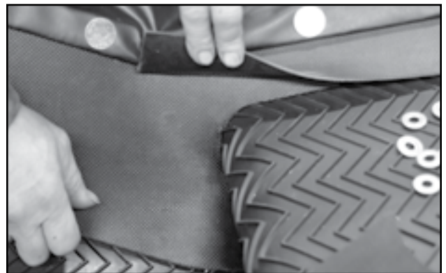
Fig 108 - Corner flashing tight around roller
