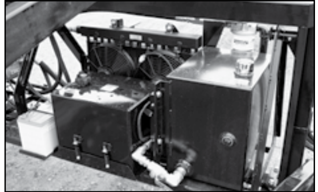
Fig 61 - Hydraulic oil reservoir and fuel tank
