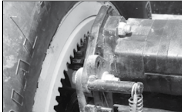
Fig 111 - Bin fill conveyor drive gears
