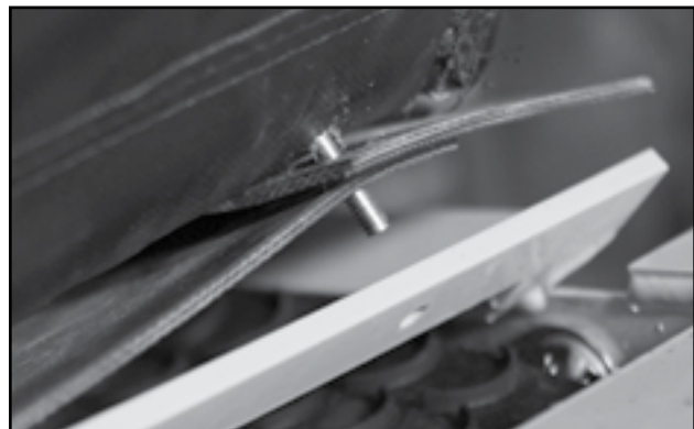
Fig 105 - Insert bolt through top, side and tail flashing
