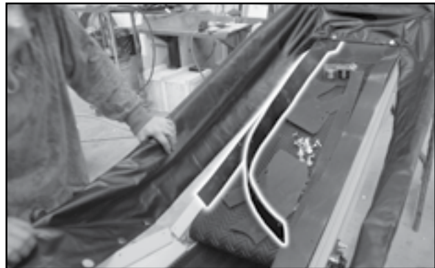
Fig 104 - Layer side flashing pieces
