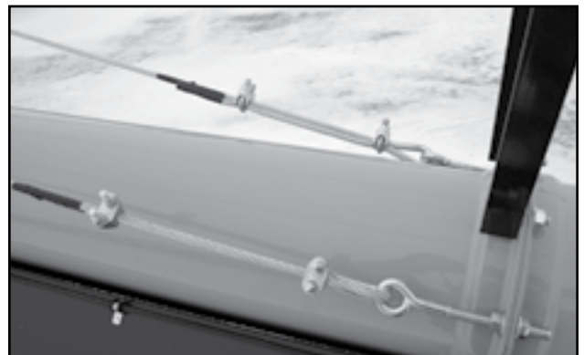
Fig 65 - Cable bridging eye bolts
