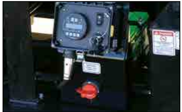
Fig 38 - Engine control and battery lock-out
