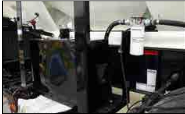
Fig 70 - Hydraulic reservoir and filter
