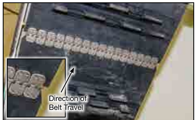
Fig 69 - Alligator lacing on rear conveyor paddle belt
