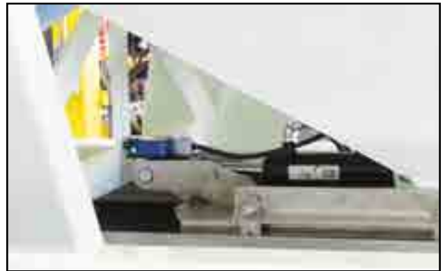
Fig 46 - Compartment gate cylinder
