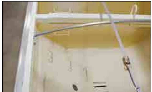
Fig 28 - Compartment ladder rungs
