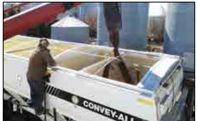
Fig 40 - Transporting CST to site
