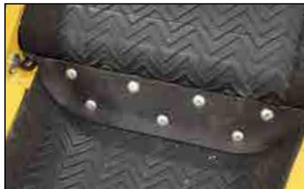
Fig 100 - Transition Flashing in place
