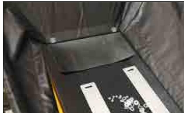
Fig 92 - Tail flashing on top of side flashing
