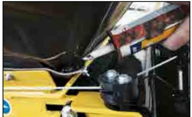
Fig 111 - Silicone gap in front corners
