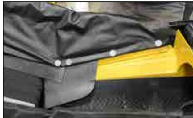
Fig 93 - Transition corner flashing in place
