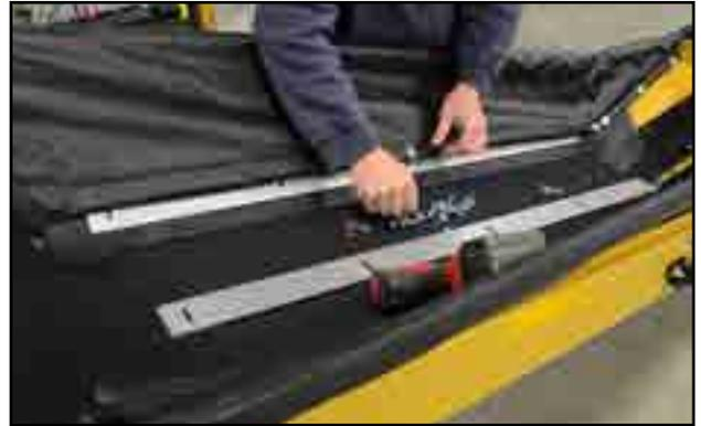
Fig 94 - Stainless steel flat bar to hold side flashing
