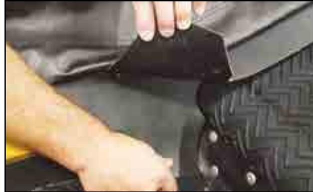
Fig 105 - Corner flashing against roller
