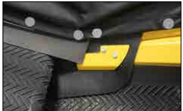
Fig 96 - Fasten flashing clamp
