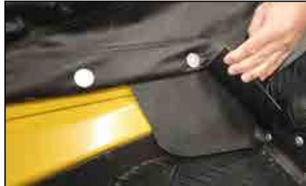
Fig 106 - Flashing fastened along transition
