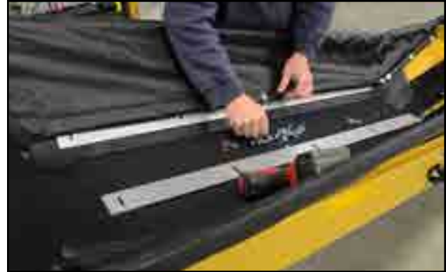
Fig 67 - Stainless steel flat bar to hold side flashing
