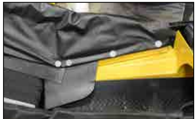
Fig 65 - Transition corner flashing in place
