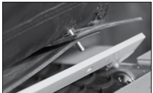
Fig 78 - Insert bolt through top, side and tail flashing
