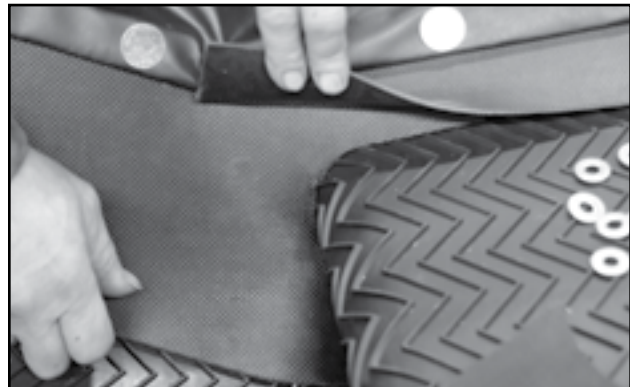
Fig 81 - Corner flashing tight around roller
