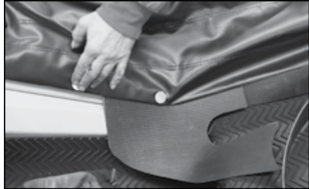
Fig 79 - Corner flashing
