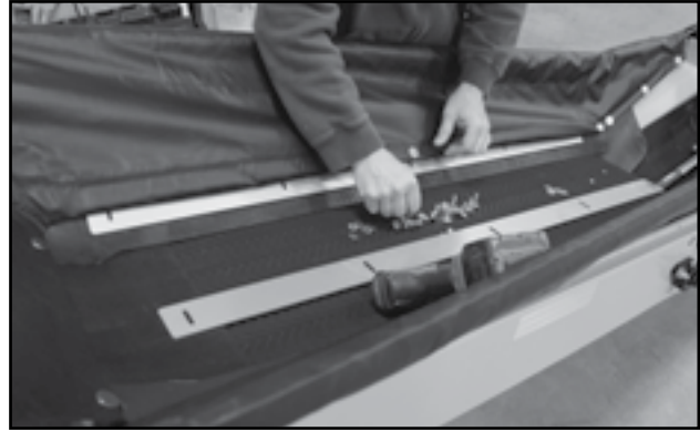
Fig 79 - Stainless steel flat bar to hold side flashing
