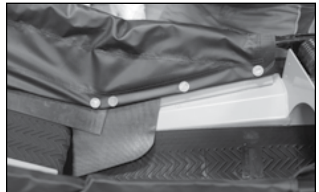
Fig 78 - Transition corner flashing in place
