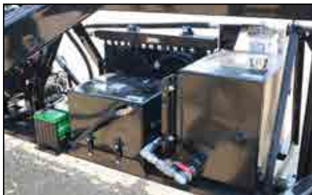
Fig 62 - Hydraulic oil reservoir and fuel tank
