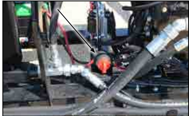
Fig 9 - Power shut-off switch
