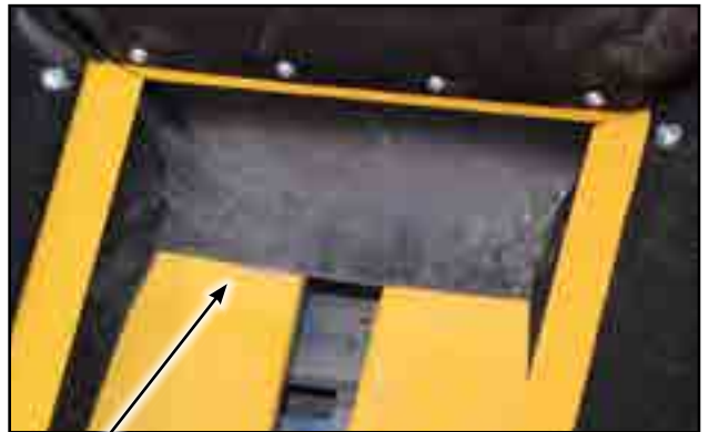
Fig 99 - New tail flashing
