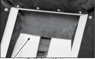
Fig 99 - New tail flashing
