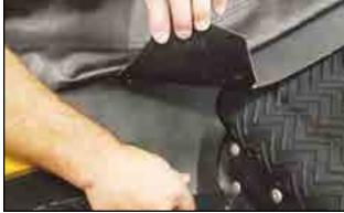
Fig 105 - Corner flashing against roller
