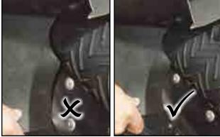
Fig 109 - Corner flashing must fit tight
